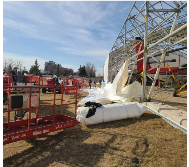
Tent hangar reskinning
