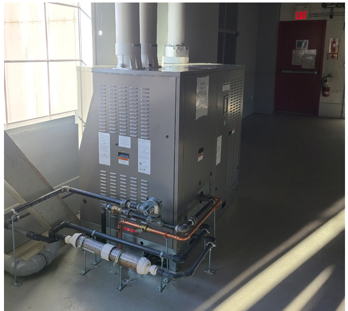
A new humidity system installed in our Main Hangar
